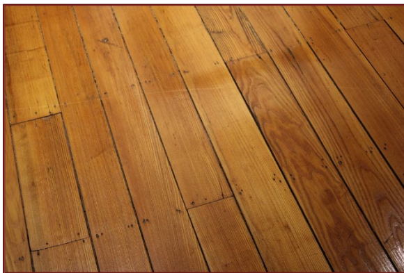
Figure 4-30. Original wood flooring in Room 1-7, 2025.
