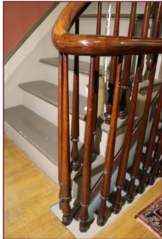
Figure 4-37. Balustrade, Room 2-2, Identical to that in Room 1-2, 2025.
