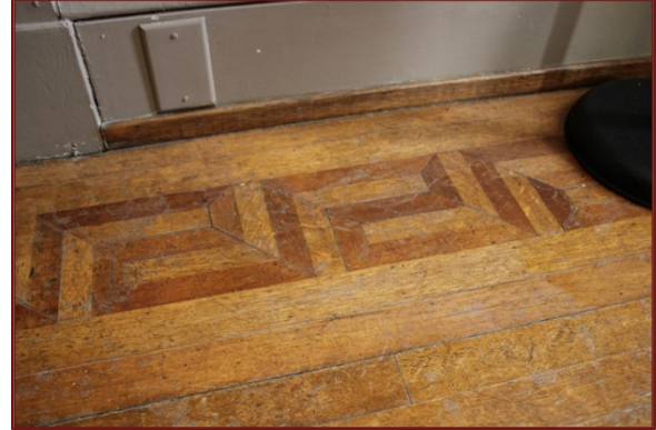
Figure 4-18. Greek key floor detailing and simple baseboard trim, in Room 1-2, 2025.
