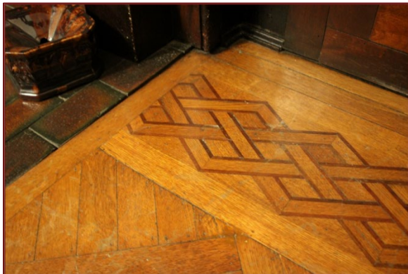
Figure 4-27. Oak flooring with Greek Key detail in Room 1-1, 2025.
