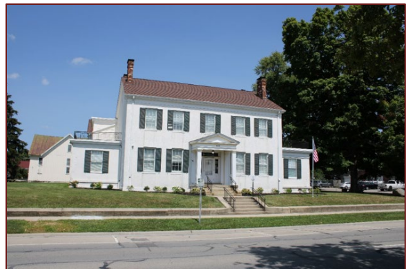
Figure 4-2. Rombach Place 2024, main (south) facade showing proximity to the street, facing northeast, 2024.
