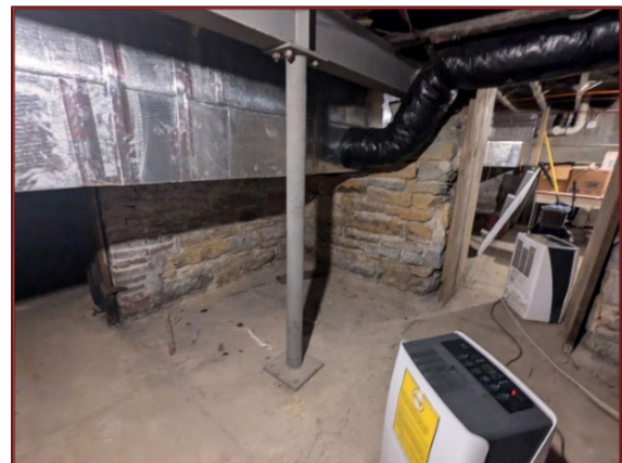
Figure 4-56. Basement western room, 2024.
