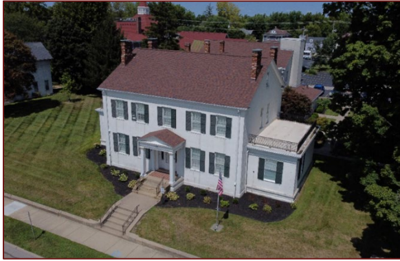
Figure 4-1. Rombach Place 2024, primary (south) facade, facing northwest, 2024.
