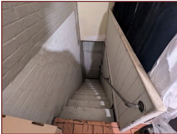
Figure 4-50. Disused staircase in Room 2-9, 2024.
