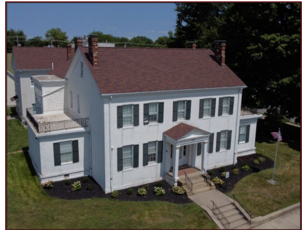
Figure 3-1. West and primary (south) facade of Rombach Place, facing northeast, 2024.
