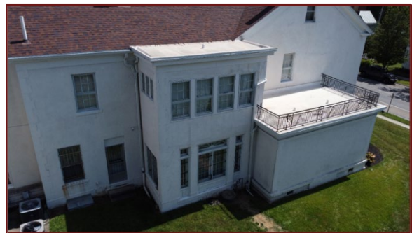
Figure 4-11. Rombach Place (2024), east and north facades, facing southeast, 2024.
