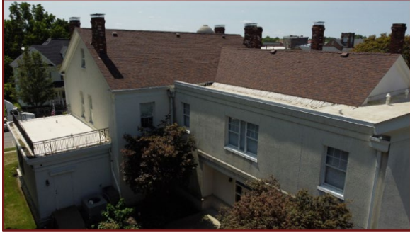
Figure 4-12. Rombach Place (2024), east facade, partially occluded by vegetation, facing southwest, 2024.
