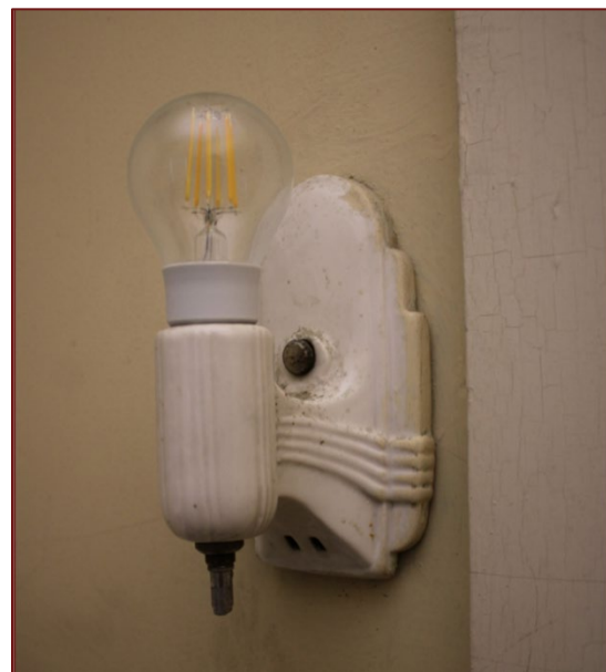
Figure 4-49. Extant Art Deco porcelain lighting sconce in Room 2-8, 2025.
