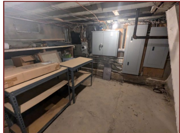
Figure 4-55. Basement main room, 2024.
