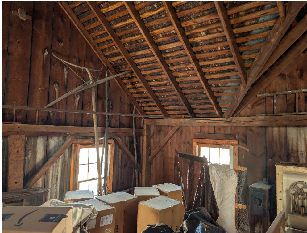
Figure 4-15 Overview of Second Floor, facing NW, 2024
