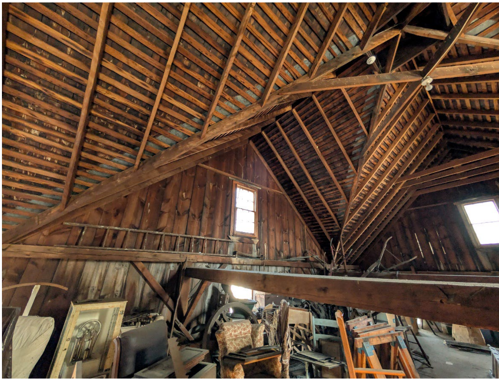
Figure 4-17 Overview of Second Floor, facing NE, 2024
