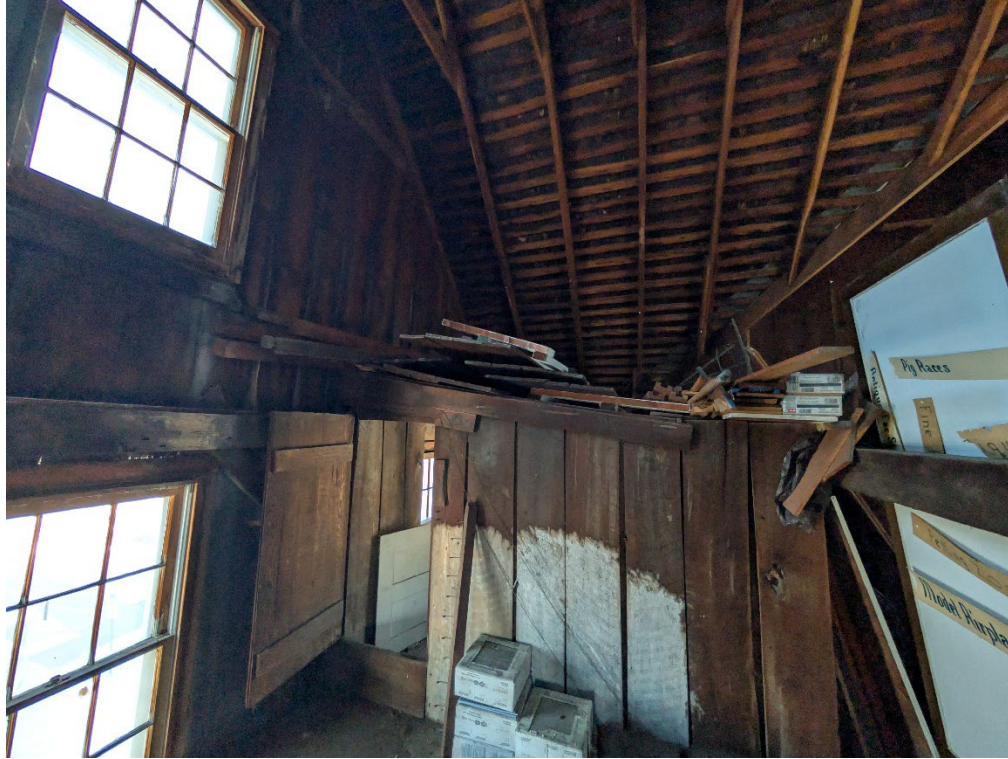
Figure 4-18 Overview of Small Room, Second Floor, facing SE, 2024
