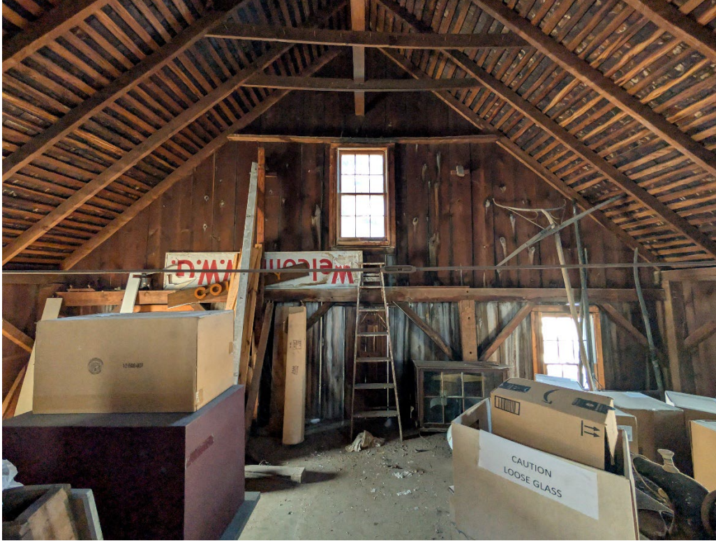
Figure 4-16 Overview of Second Floor, facing W, 2024
