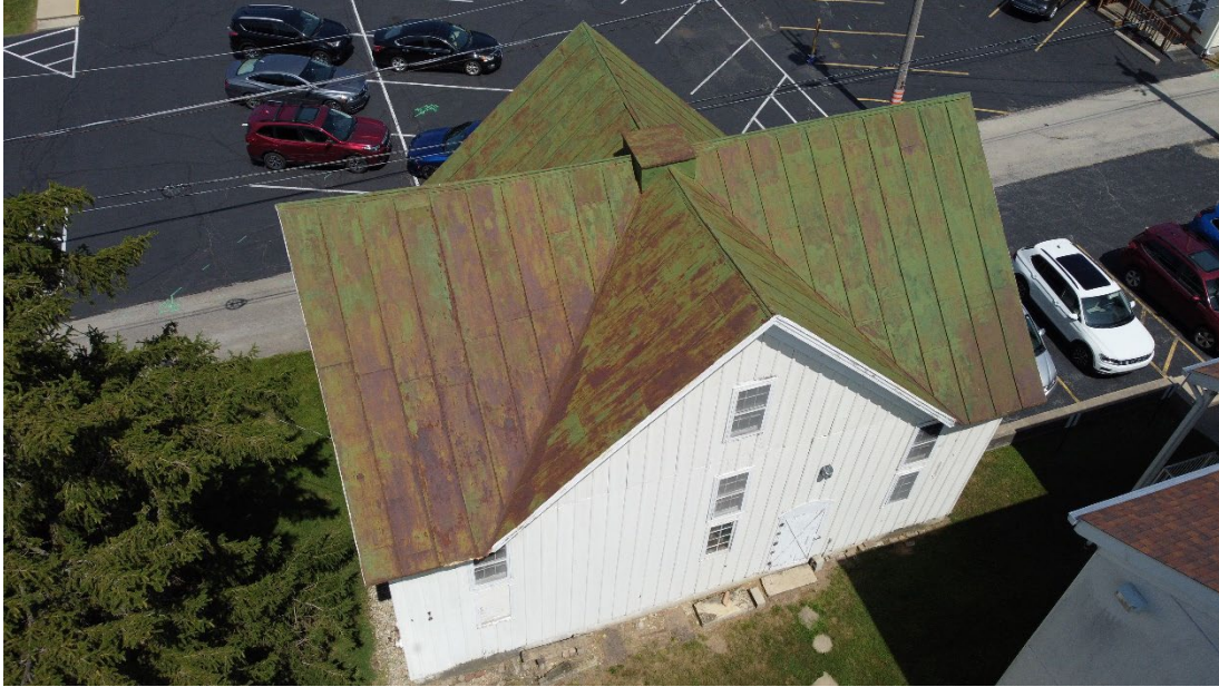
Figure 4-1 Photograph of Carriage House, south (main) façade and roof, facing northeast, 2024
